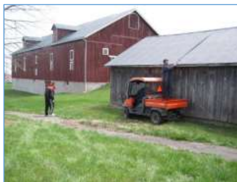
Fixing the Shed Roof
